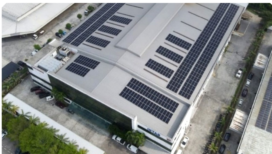
Solar PV system at MTAG Group's main plant in Tebrau
